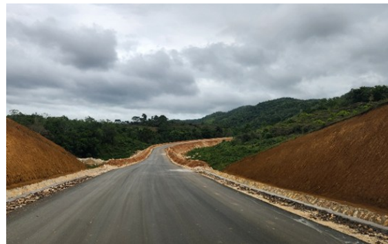
Figure 3 and 4: Haul road construction by Winalco to Penny
